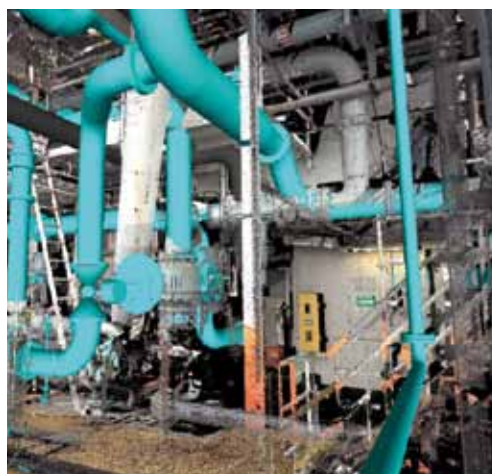
3D point clouds of offshore installations.
