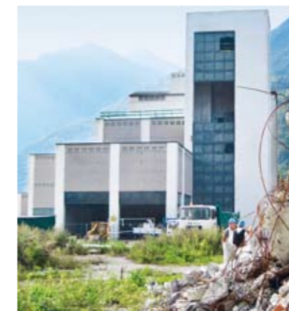
Ramboll was the Client's Representative at the waste-to-energy facility in the Isle of Man and is now assisting the Isle of Man government during its 25-year operation contract with the operator.
